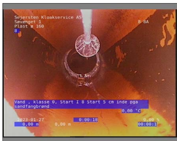
Foto: 28_1_1_27012023_102407_1.JPG 0m, Vand, klasse 0 / Start I 8 Start 5 cm inde pga sandfangbrønd
